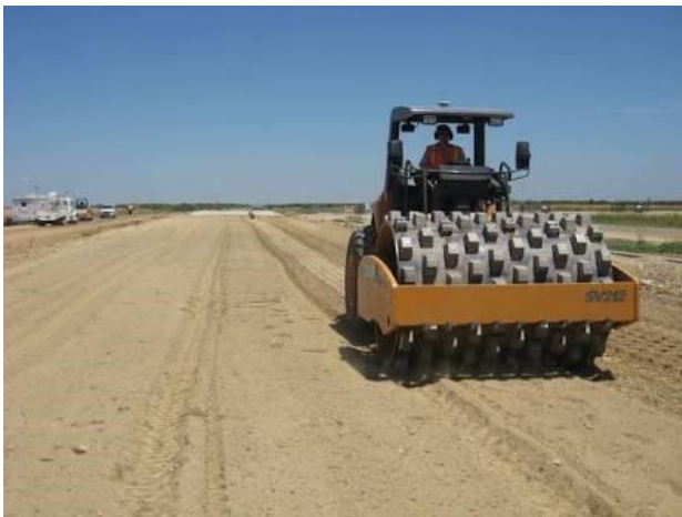
Fig No. 3 soil stabilization using sheep foot roller and rammer
