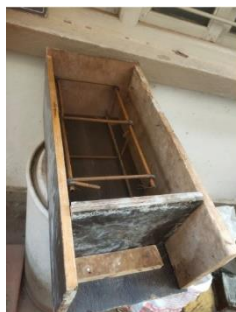
fig.3 Mould for column
