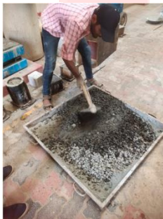
Fig.2 Concrete Mixing process
