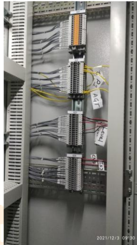
Figure 3. I/O's connection at DCS coming from loop
