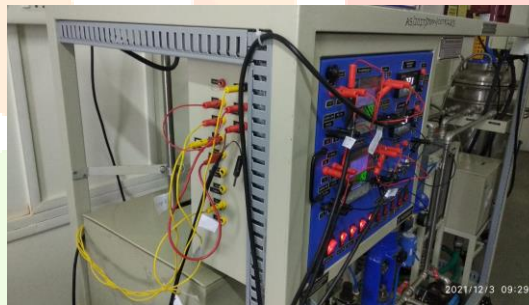
Figure 4. I/O's connection at loop coming from DCS.
