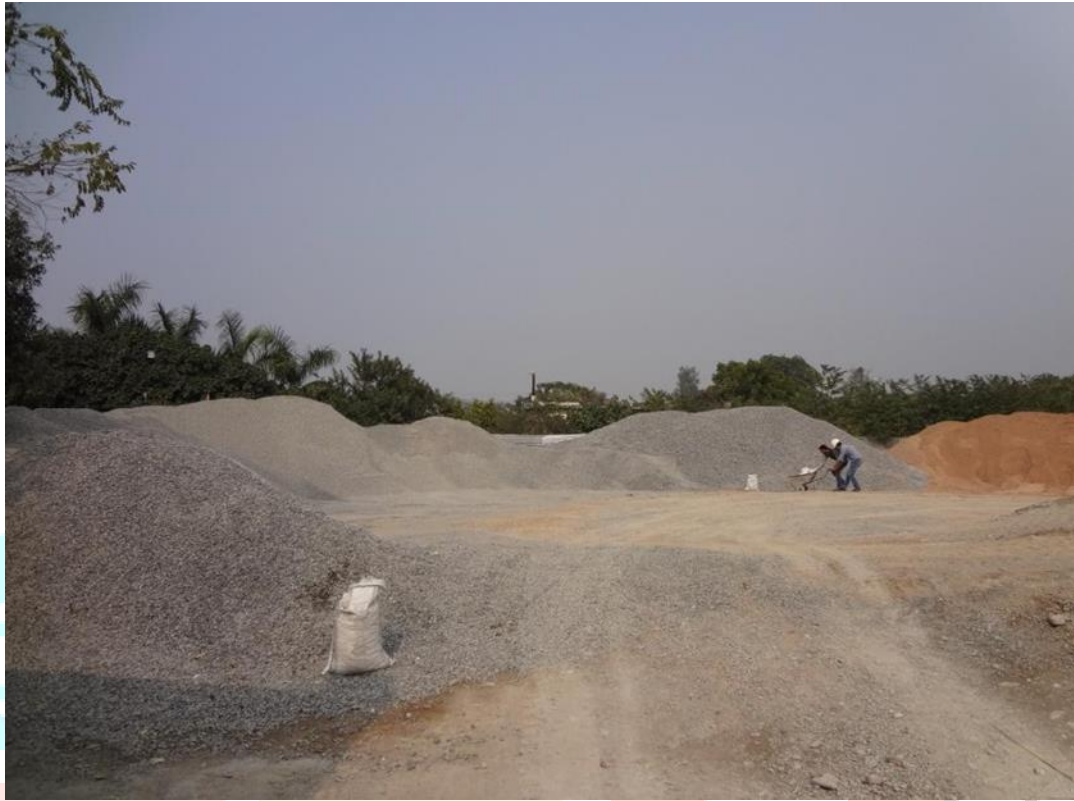
Fig: 1.2 Aggregate in open field
