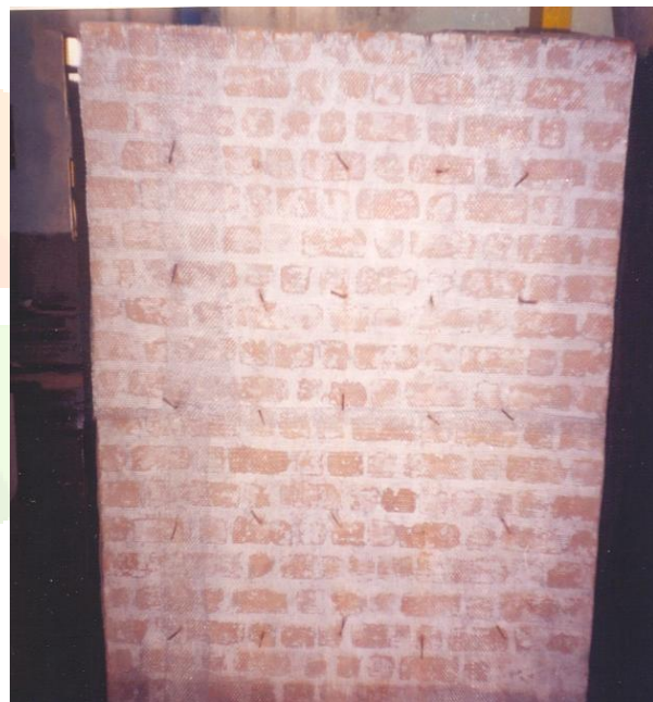
Plate 2 Fixing of wire mesh with M.S. rods and nails.
