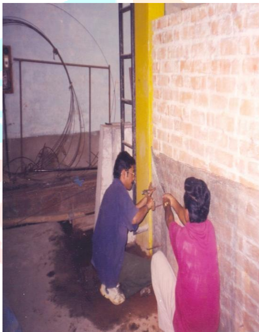
Plate 1 Fixing of wire mesh to wall With nails only.
