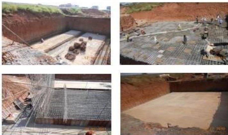
Fig-2 Construction of Thrust Bed
