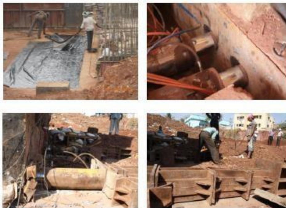
FIG-3: PUSHING BOX SEGMENTS USING HYDRAULIC JACK
