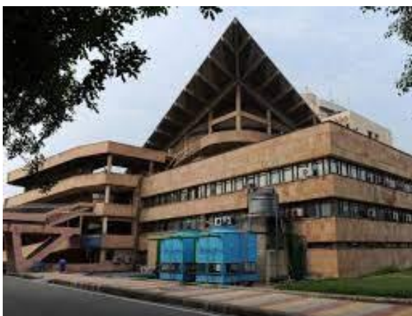
Fig. 1.3 Front View of Centre of Excellence for the renewable energy in the campus of IIT Delhi
