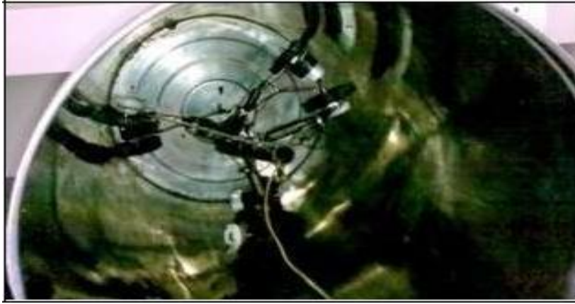
Figure.10 PIR moving inside the pipe
