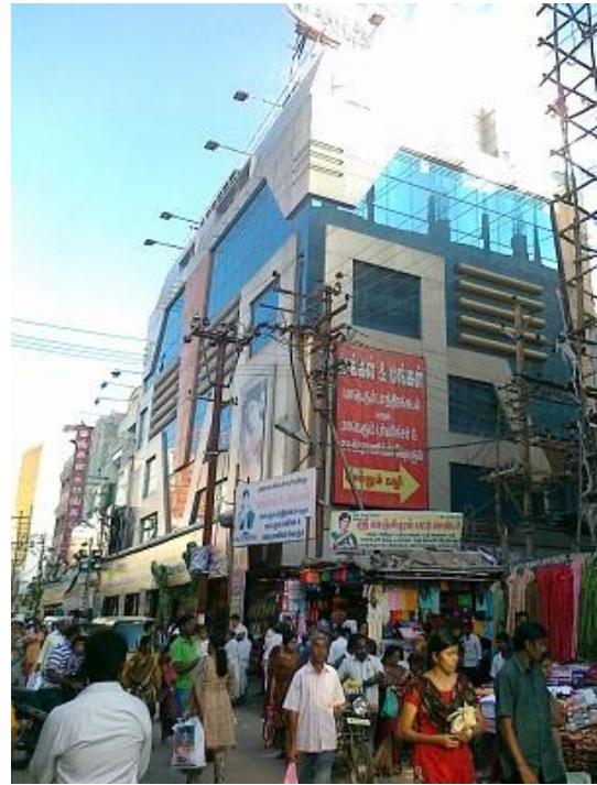
Fig.6. Shops in Rockfort area, Tiruchirappalli
