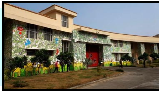
Figure 3: Madhubani Mural Art on plaster wall
