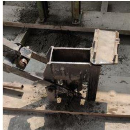
Fig 2: Mixing Cement & Sand, Water
