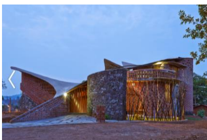
Fig-31 Showing the use of Locally available materials
