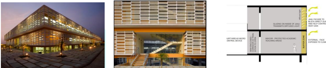
Fig-33 Showing the use of Brick jalis and Passive cooling Techniques
