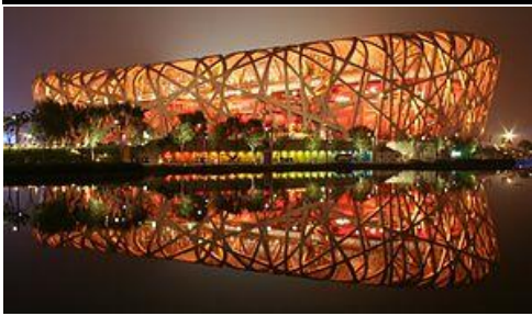
Fig-20 Bird's Nest National Stadium Beijing
