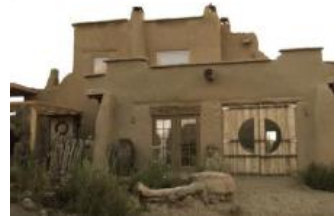
Fig-11 Adobe residence built by owner builder in USA
