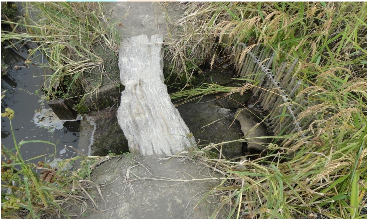
Sharing of water through ditch made up of concrete
