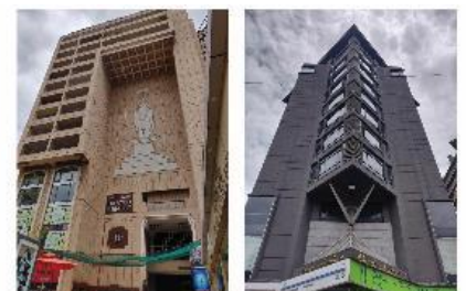
High Rise (G+15): Barton centre, Trinity Towers
