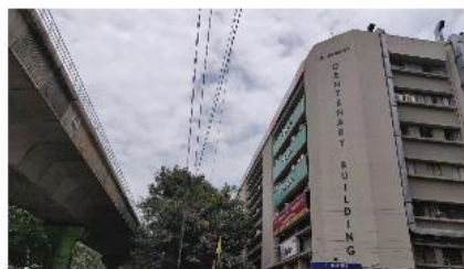
Mid Rise (G+7): Centenary Building
