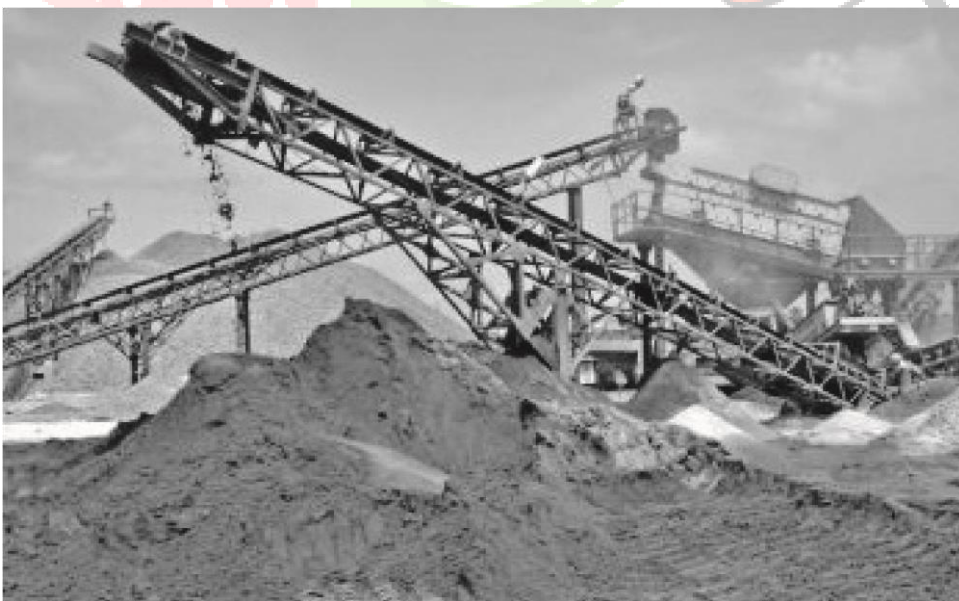
Fig. 2.2 M-sand manufacturing unit near Coimbatore (Tamil Nadu) Japanese manufacturers began, around the turn of the millennium, to seek a potential niche to fill in the quarrying market. The only growth area seemed to be in the production of
