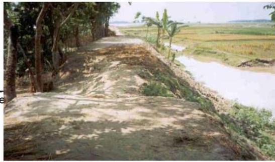
Figure-20 Settlement of Crest and side slope
