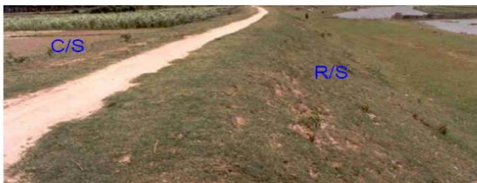
Figure-1 Flood Management Embankment
