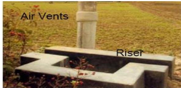
Figure-10 Air vents & Riser
