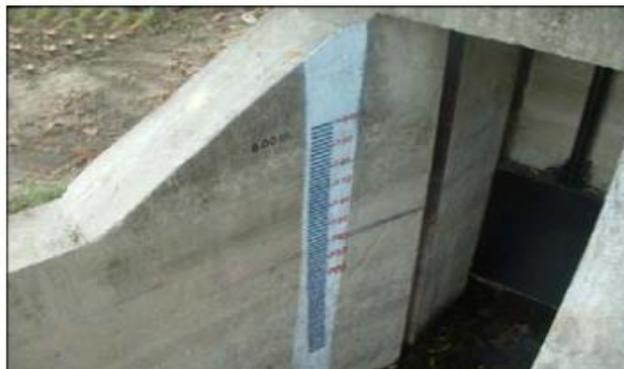
Figure-15 Water Level Gauge
