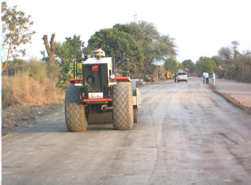
Figures 4 - Compacting By Vibrator Roller at Site.
