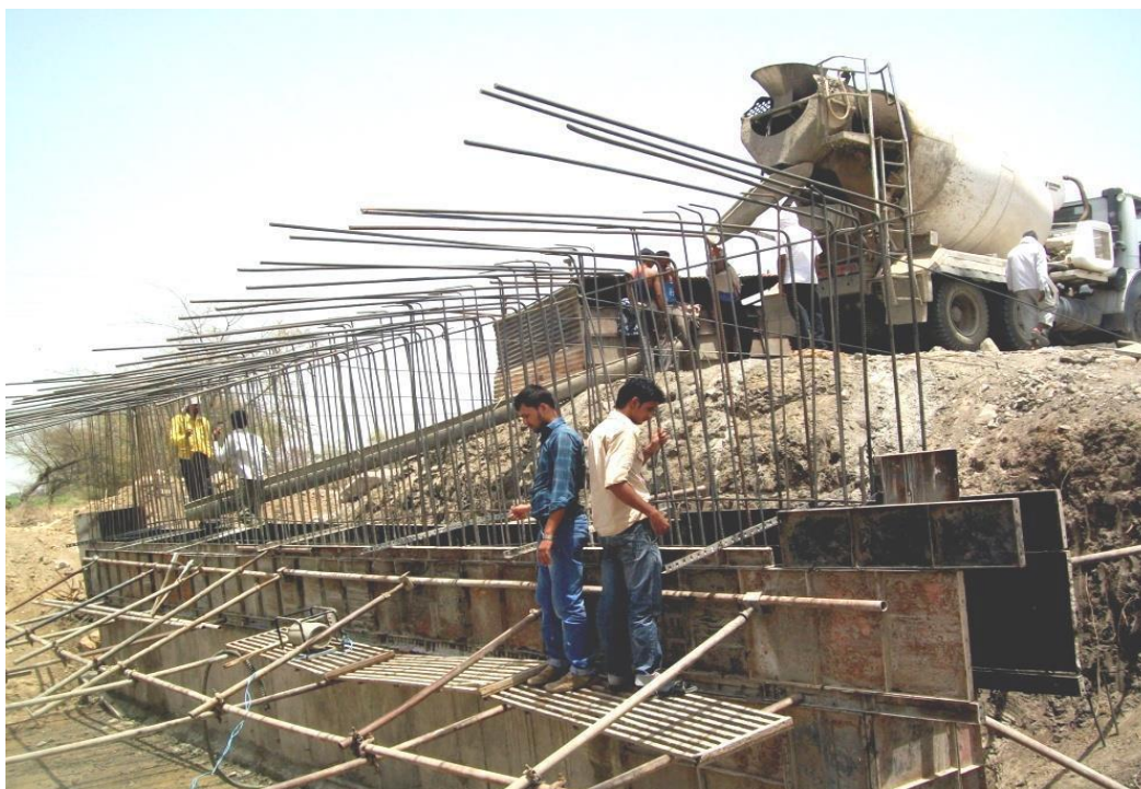
Figure 2 -concreting in box culvert at sites
