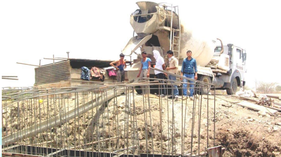
Figure 8 - Placing of Concrete through Chute by Transit Mixer
