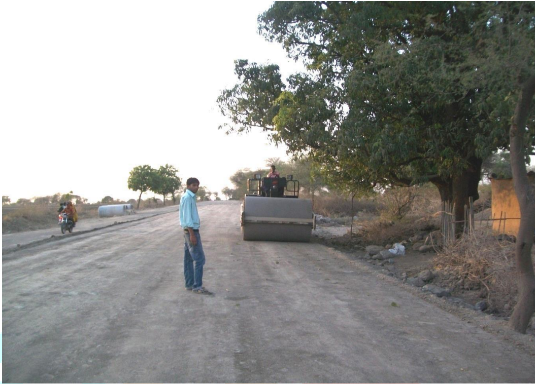
Figures 3 - Compacting By Vibrator Roller at Site.
