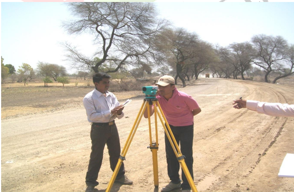
Figure 1 -Checking Level of Super Elevation
