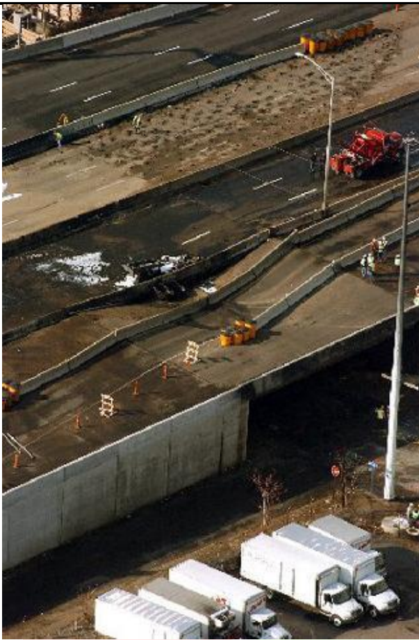
Figure 1.7. Oil Tanker Blast at Interstate.
