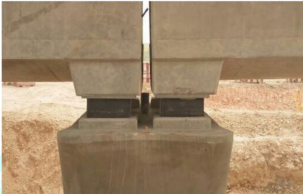
Figure 3.8. Installation of Elastomeric bridge bearing under girder.
