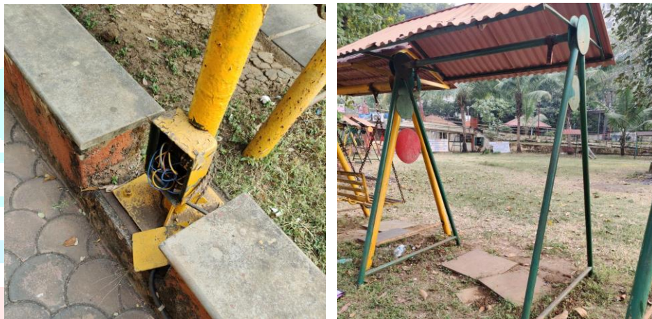
Image 13 (left) & 14 (right) - Non-maintenance of facilities & installations
