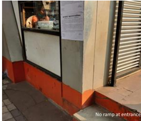
Image 12 - Inadequate provisions for universal accessibility
