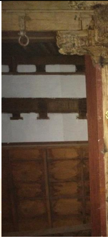
Fig 49 Bathroom steel strengthening column
