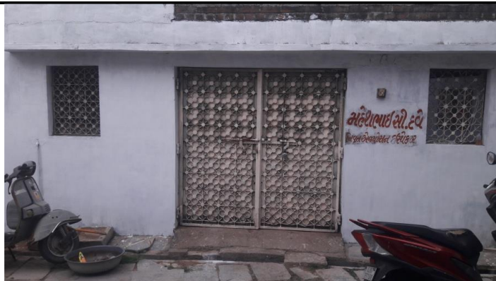
Fig 25 Timber Lime Structure
