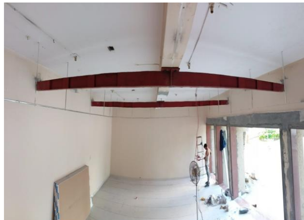
Fig 22 Two numbers of ISMB250 at APC
