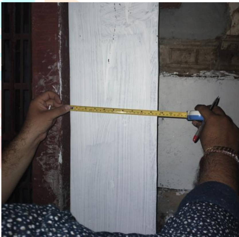
Fig 52 Measurement and site visit
