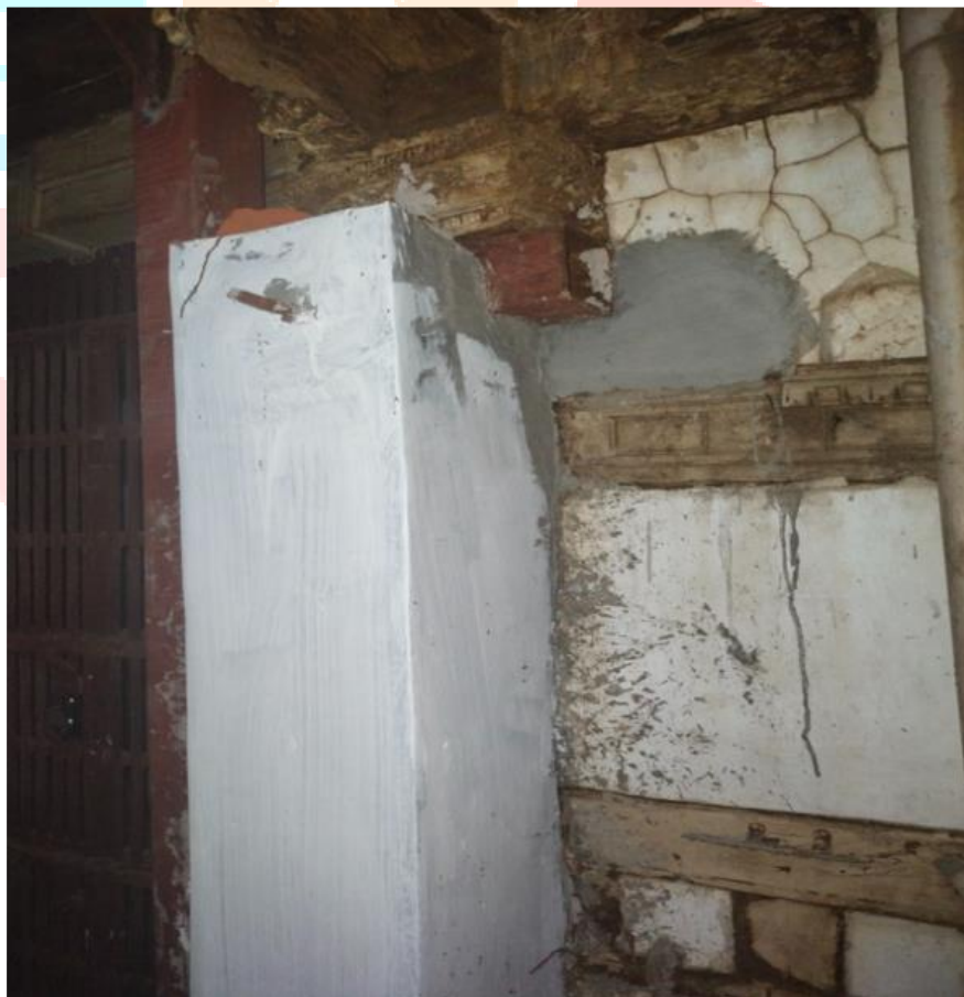
Fig 48 Kitchen cum bed room steel strengthening column
