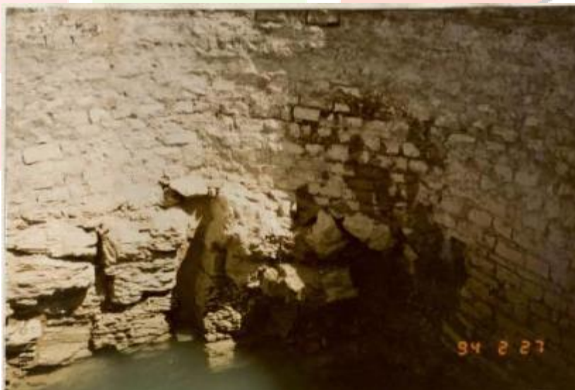
Fig. 4 Un-confined aquifer with typical dug well at village: Tohra
