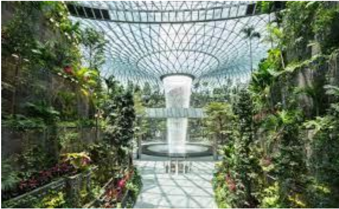
Fig.1 Rain water harvesting structure at JEWEL CHANGI, Singapore airport
