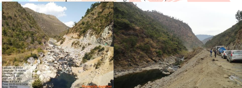
Plate 7: Debris dumped near the slope of the road, which is blocking the river (source: field survey)
