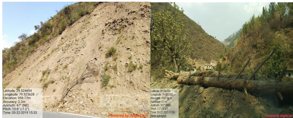
Plate 6: Effect of road widening on vegetation (source: field survey)
