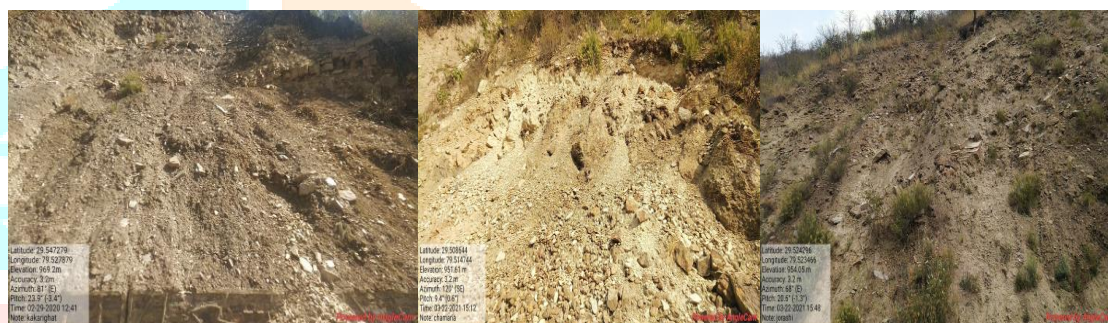
Plate 9: New landslide area (source: field survey)
