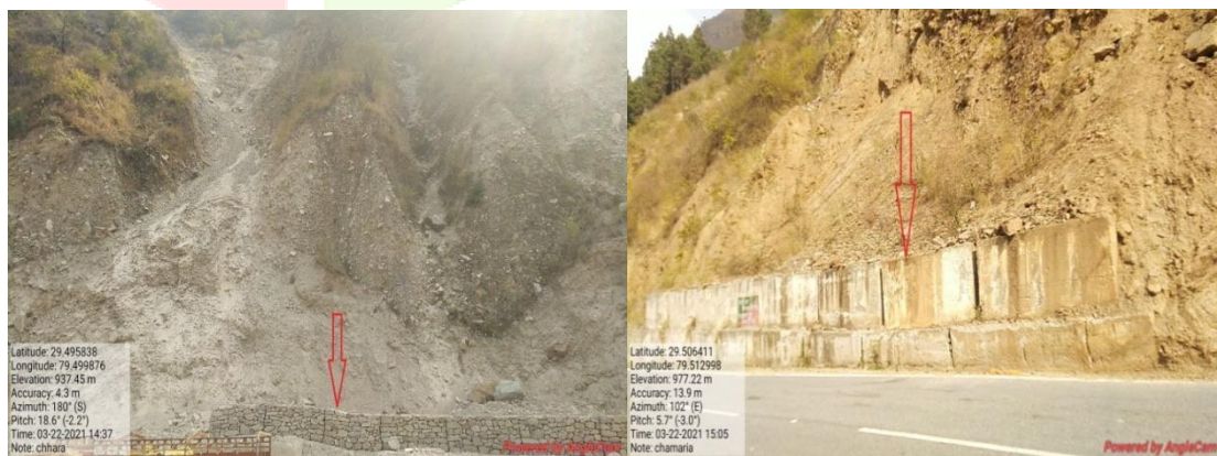
Plate 4: Concrete blocker (source: field survey)
