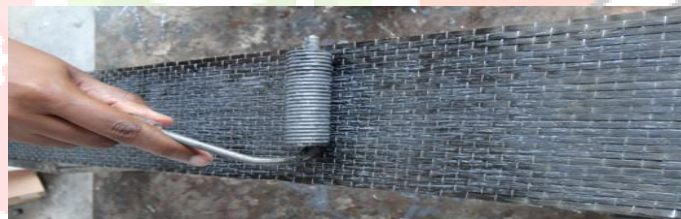
Figure 3.3 Bonding between RC beam and CFRP using Laminating Roller
