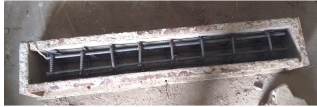
Figure 3.1 Reinforcement in Steel Moulds
