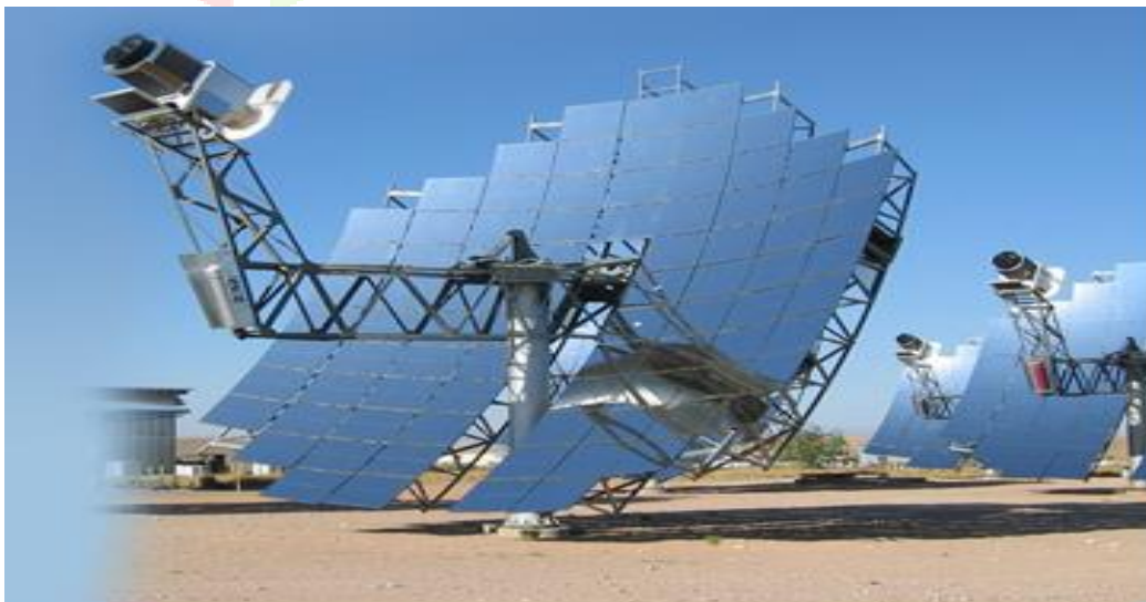
Fig. 3 A Parabolic Dish Collectors
