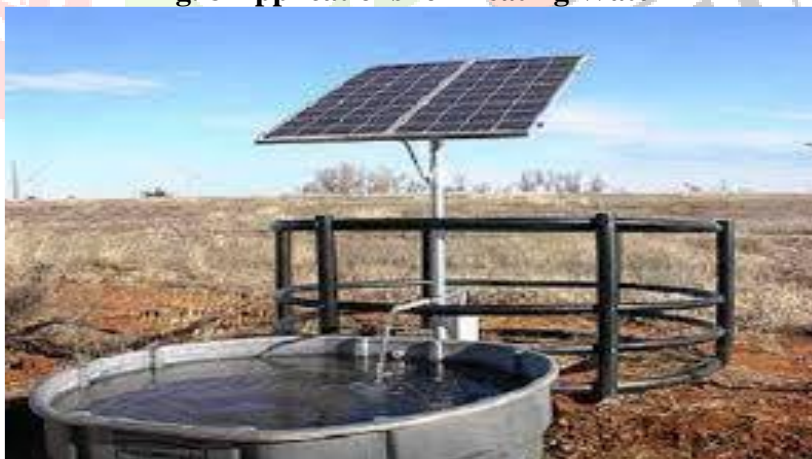
Fig. 9 Application for Water pumping
