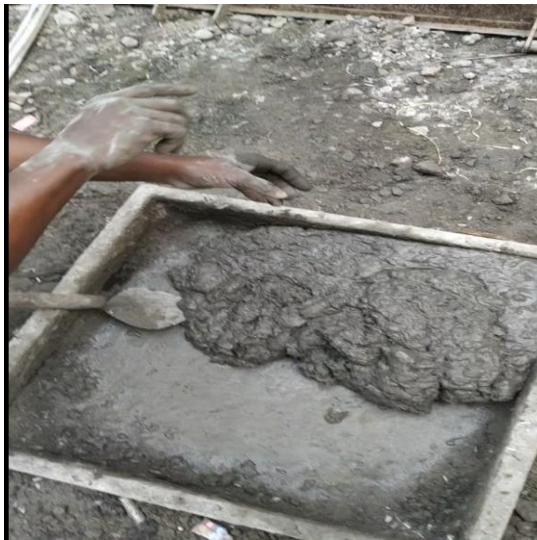
Figure Error! No text of specified style in document..6 Concrete Mixture of ECC
