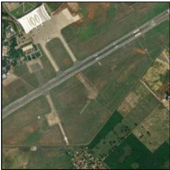
Raipur Airport View
