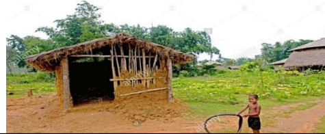
Fig V.2.4 Bamboo reinforced house with mud
