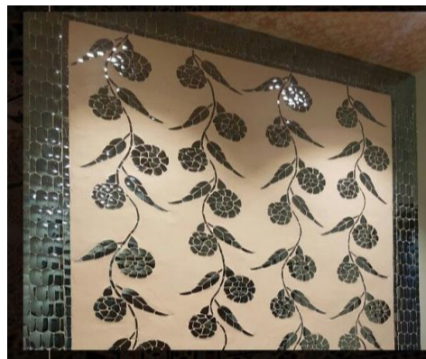
Thikri work on wall
