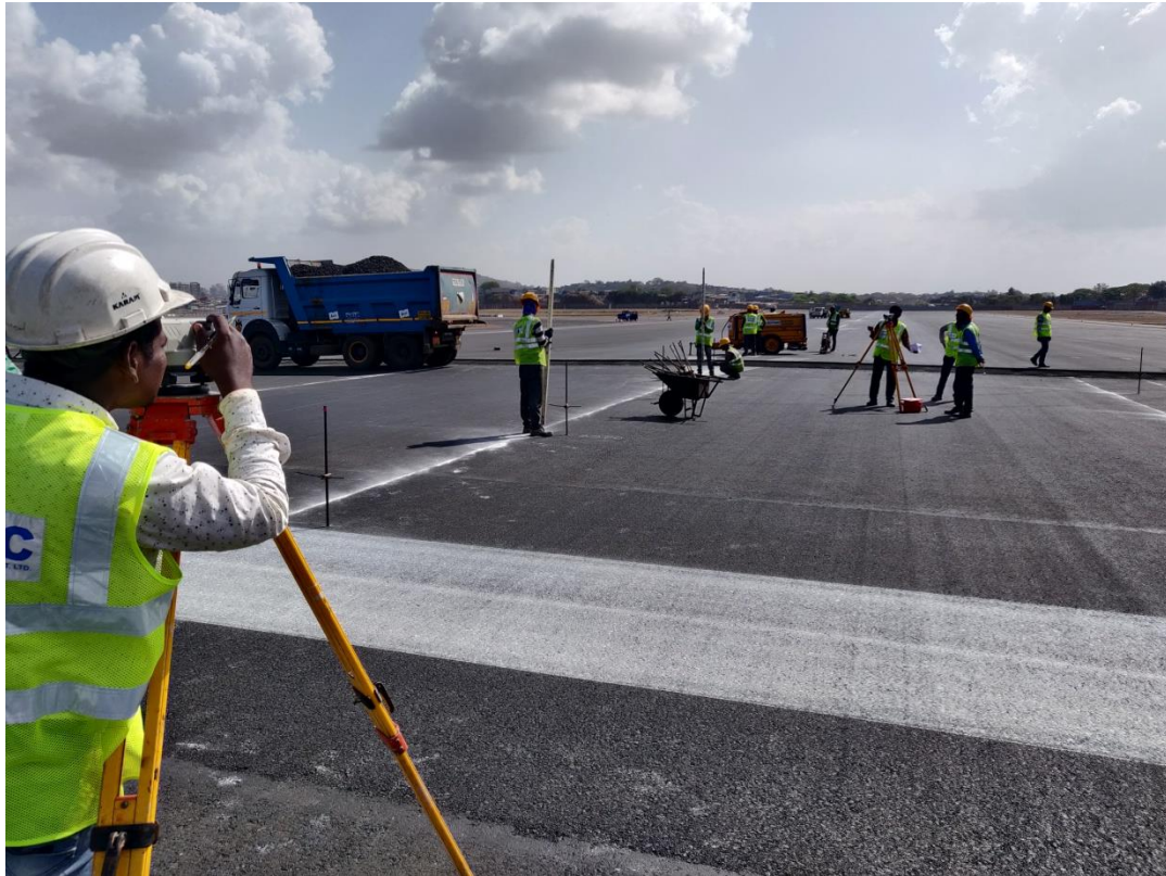
Figure 26 : Level check and fixing a point
