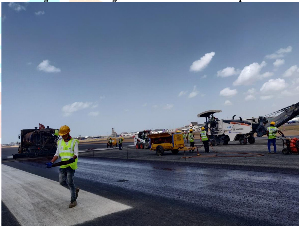
Figure 18 : Applying Tack Coat On The Milled Surface
