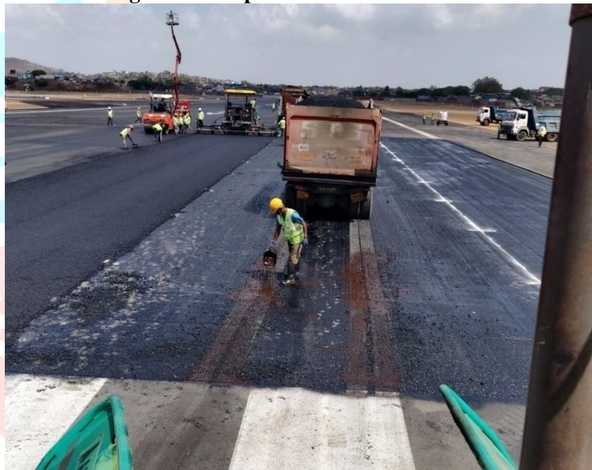
Figure 14 : Applying Tack Coat One Wheel Markings
