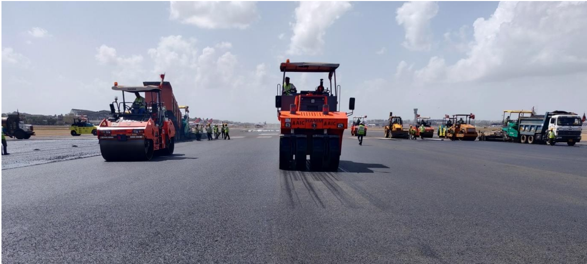
Figure 23 : Compacting The Pavement By Pnenumatic Roller
