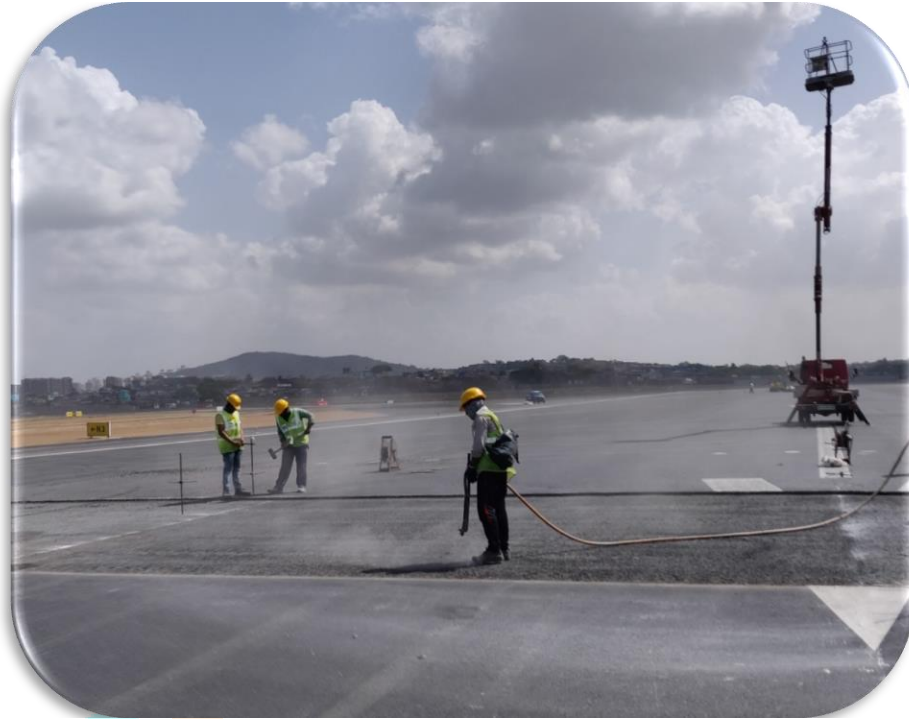
Figure 17 : Cleaning The Milled Surface With Compressor
