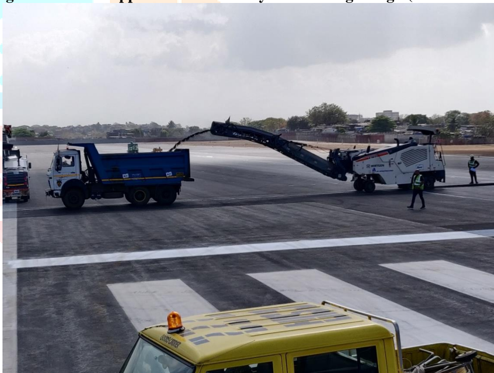
Figure 12 : Milling And Transporting Milled Material For Recycle
