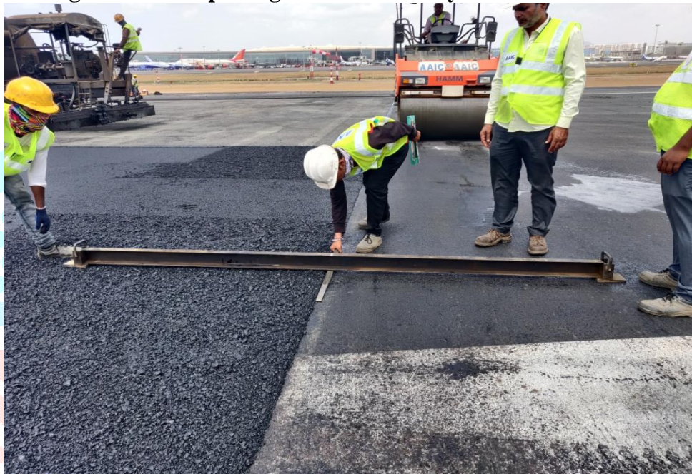
Figure 24 : Undulations are Measuring by Straightedge Test
