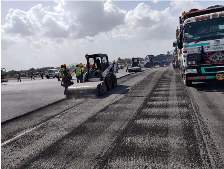
Figure 15 : Cleaning The Milled Surface With Bobcat
