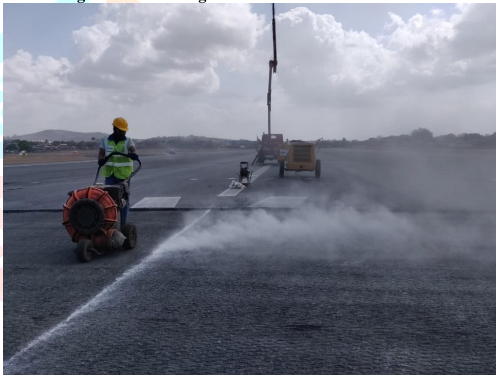
Figure 16 : Cleaning The Milled Surface With Blower
