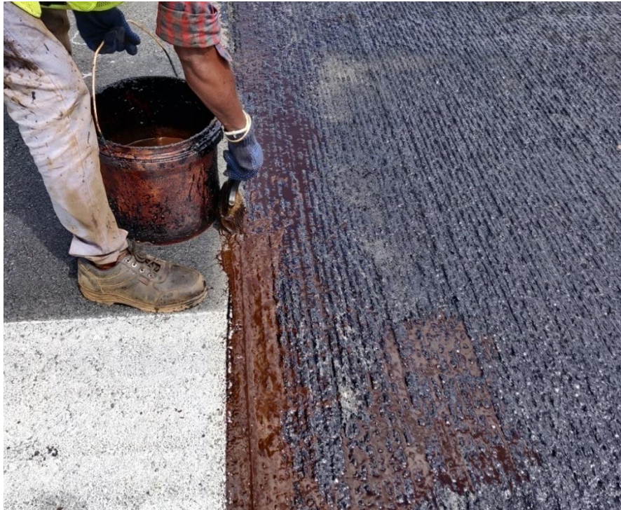
Figure 19 : Applying Brush Tack Coat On The Pavement Edge
