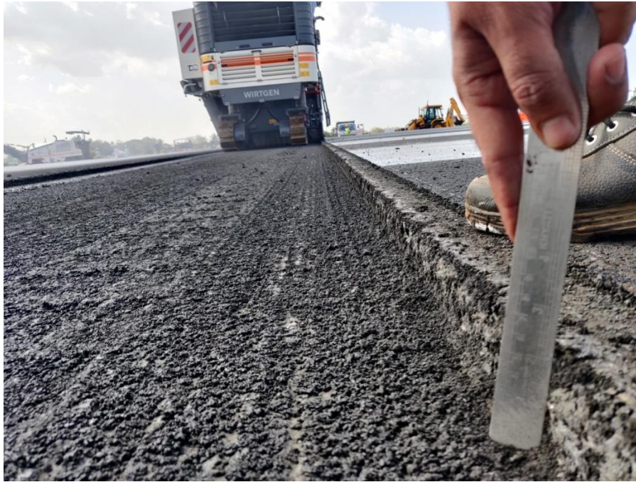
Figure 13 : Depth Check Of Milled Area
