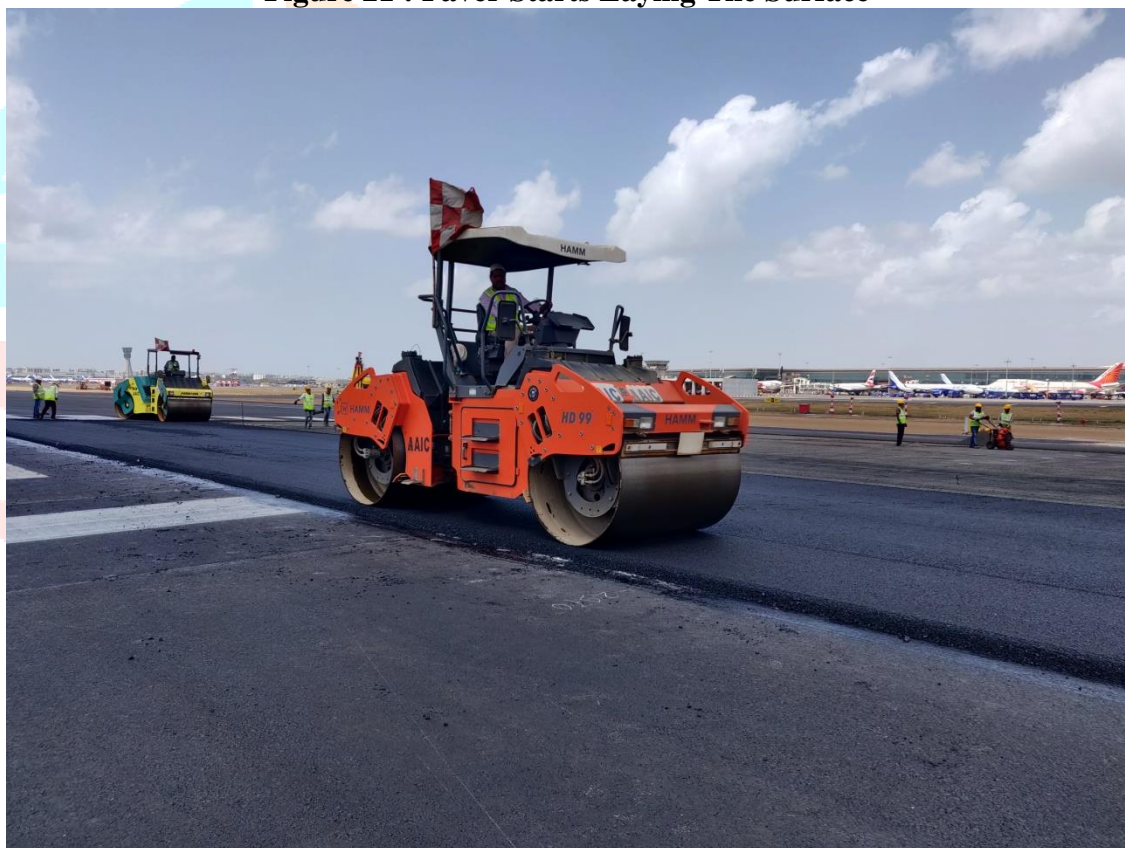
Figure 22 : Compacting The Pavement By Tandem Roller
