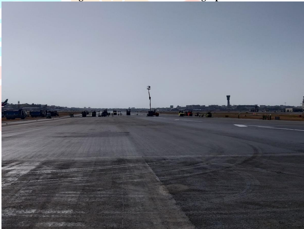
Figure 27 : New re-carpeted Runway pavement
