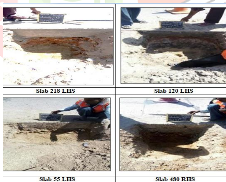
Figure 5.1: Photos of test pit
