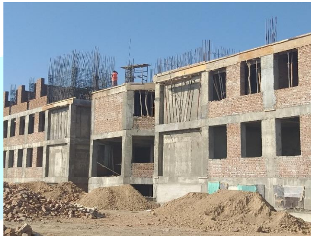
East Zone Hospital
