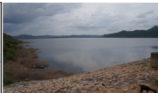
Fig. b: Large view of the Phulwaria dam at sampling site.
