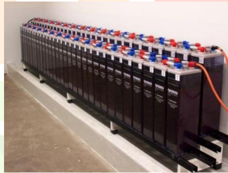
Fig 3. Battery Bank
