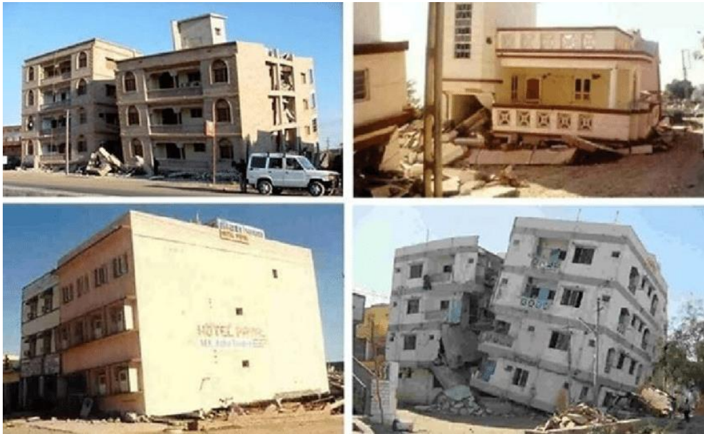
Figure 1 Damages to open/weak/soft storeys due to earthquakes Source: (Khan & Rawat, 2016)
