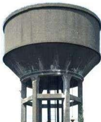
Fig 1 Intze type water tank
