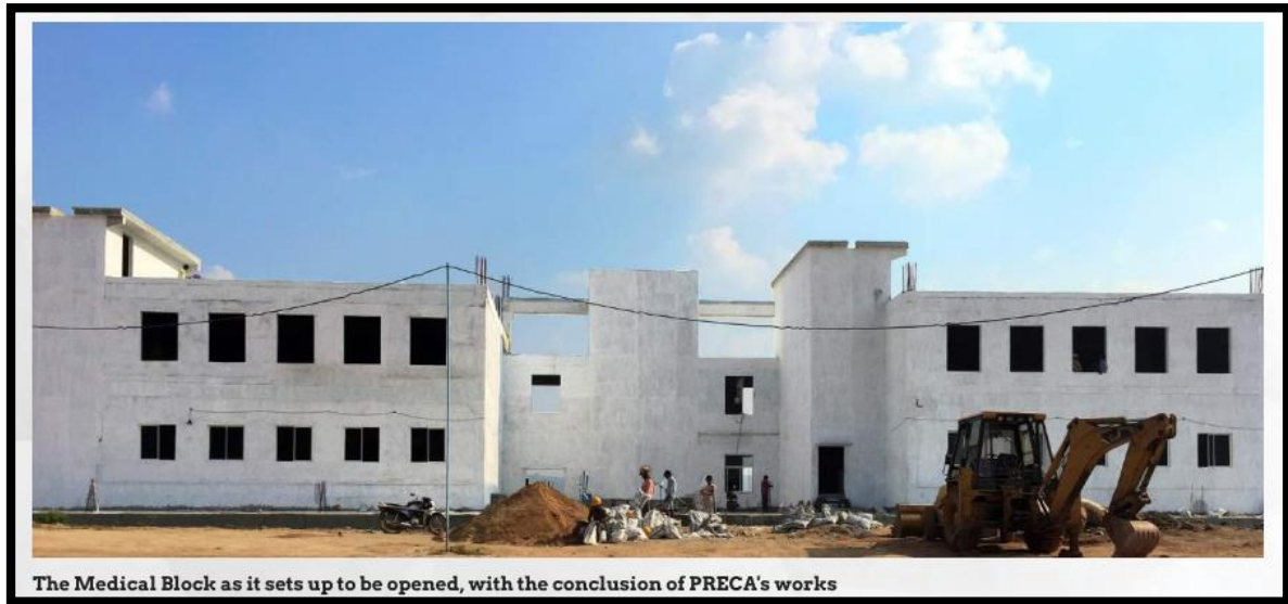
Fig 11) Building is completed using precast member [1]
