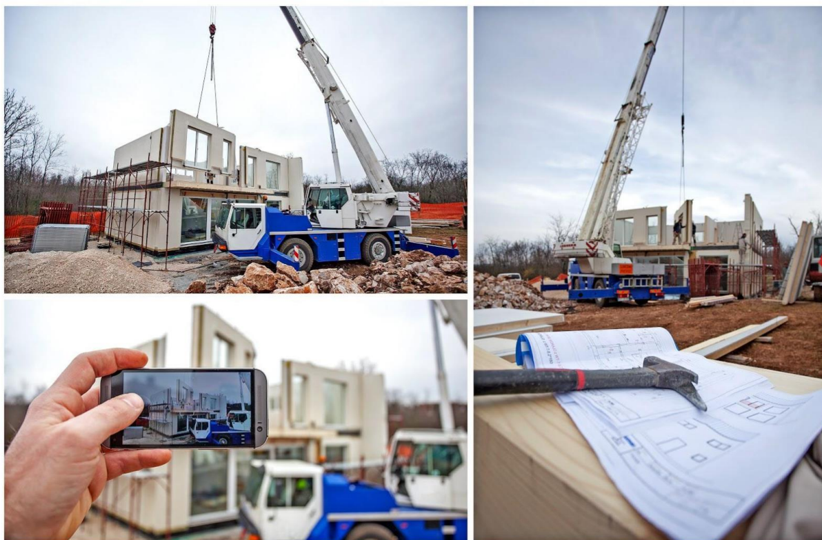
Fig.1 Typical Precast material construction [5]
