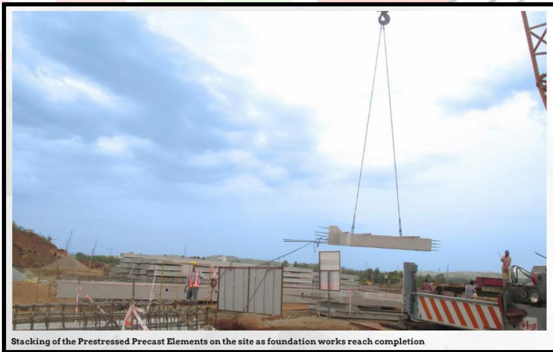
Fig. 6) Lifting of members [1]
