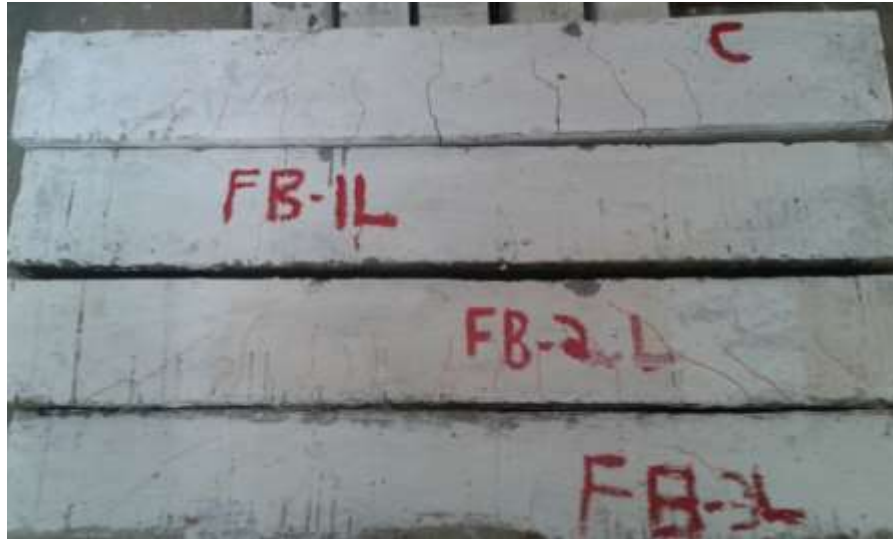
Fig.6 Crack pattern of RC all beams
