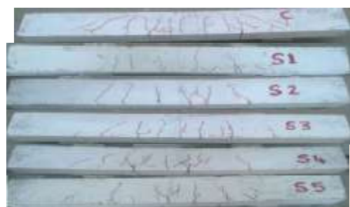
Fig.8 Failure pattern for all the beams
