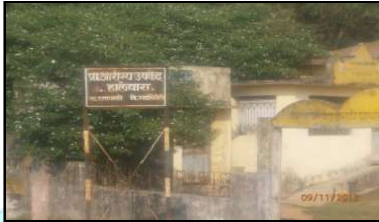
Dilapidated Status of Primary Health care centre at Halewara village of Etapalli taluka of Gadchiroli district.
