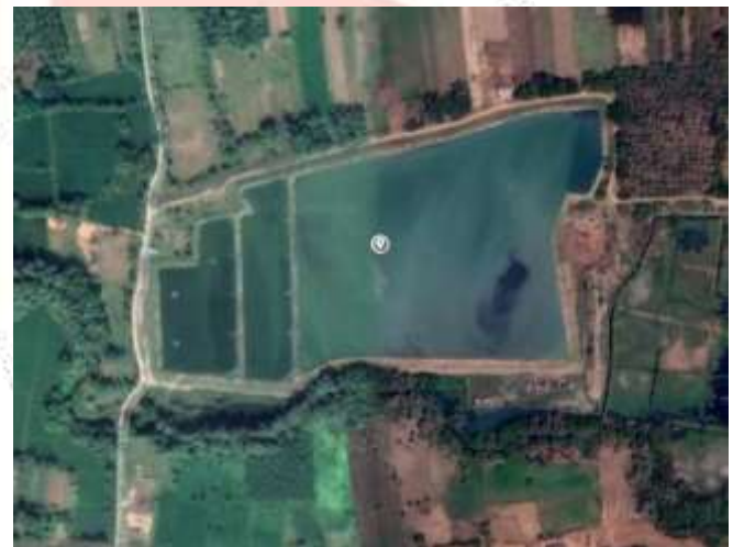
FIG (1) Shows the municipal treatment plant
