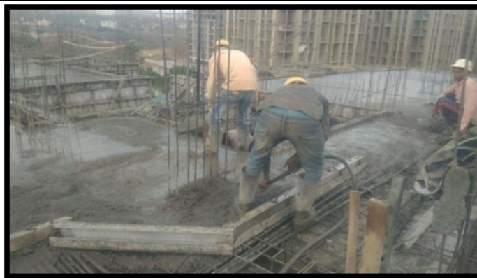
Figure 3: Monolithic slab, beam and wall casting.
