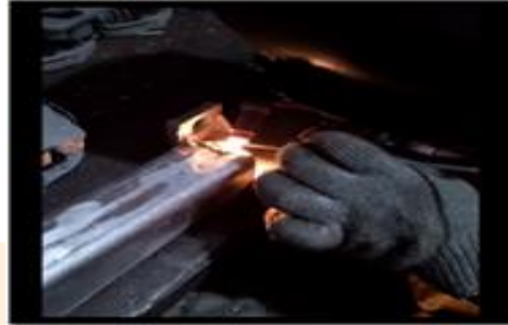
Fig.3: During the welding at defect
