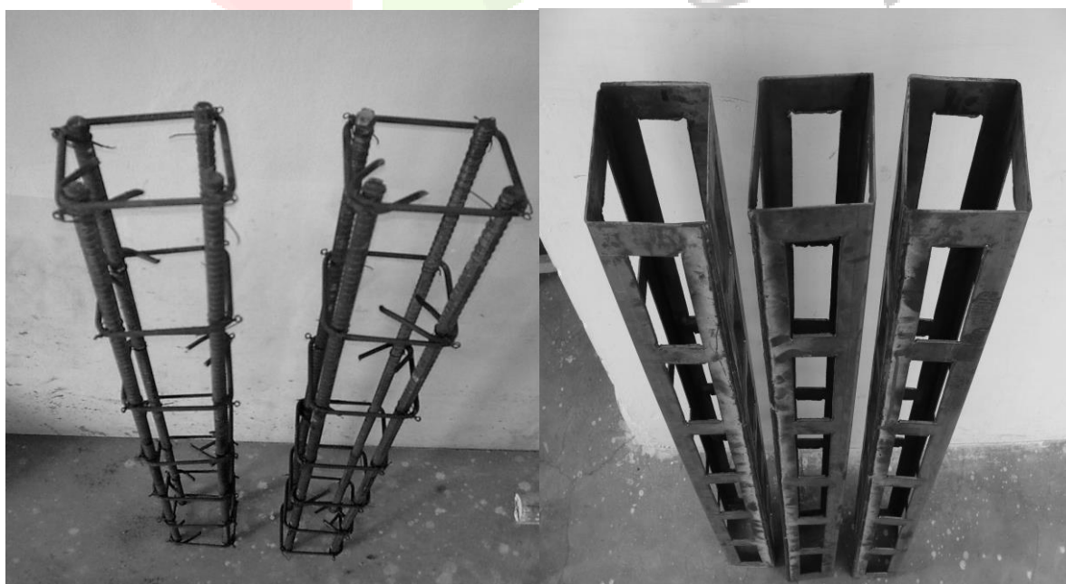
Fig.1. Rebar reinforcement and Prefabricated Cage System
