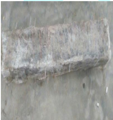
Fig no 3 Beam with GFRP wrapping
