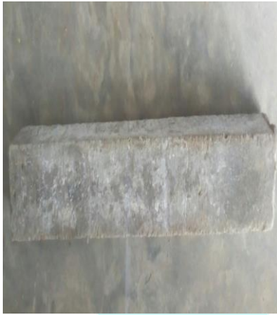
Fig no 2 Beam without GFRP wrapping
