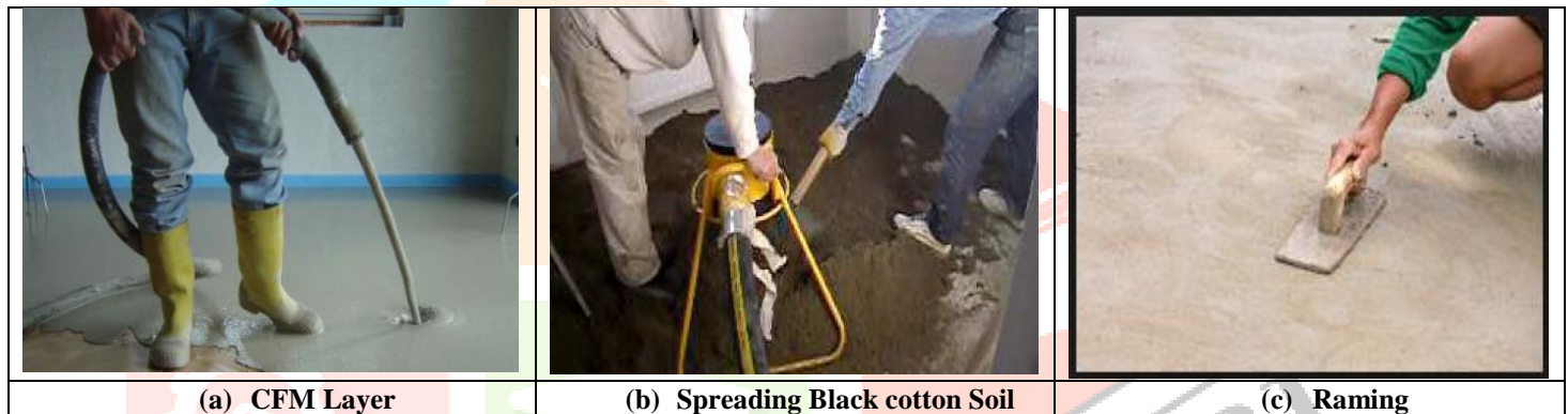
Figure 9: Floor Laying with Coir fiber mortar (with Clay soil)
