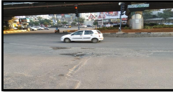
Fig 9: Potholes at the intersections causes the slow movement of the vehicles when the signal open.
