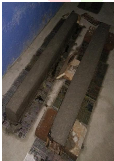
Fig 6 Casting of Beam Specimens
