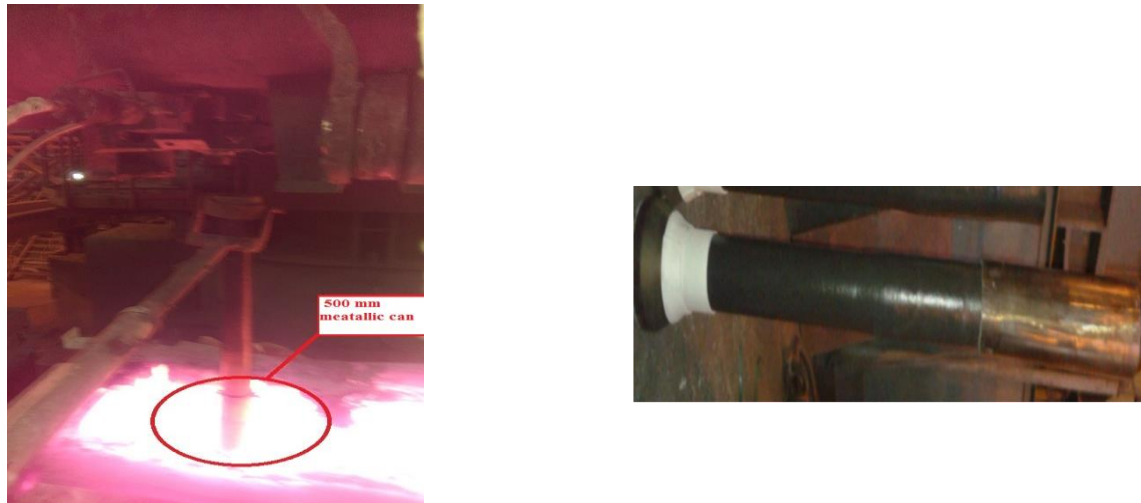
Figure-4 depicts the immersion of extended shroud to avoid emulsification in tundish.
