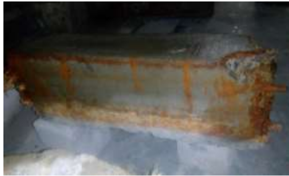
Fig.7 Corroded beam.
