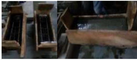
Fig.4 Moulds during casting.
