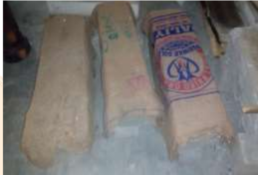
Fig.5 Curing of beams.
